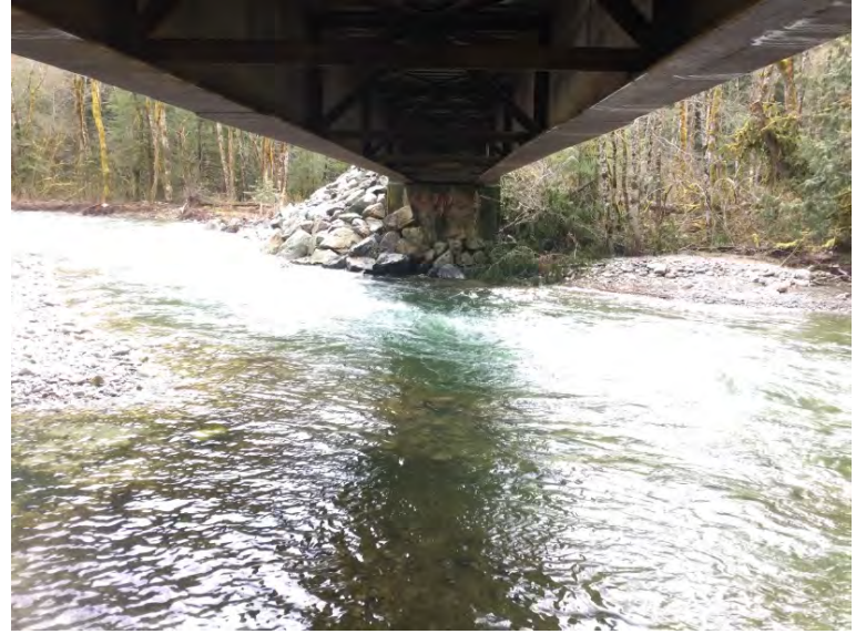
Left Bank Abutment when facing downstream
