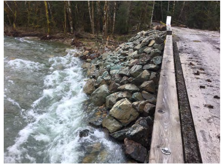
Upstream left bank riprap
