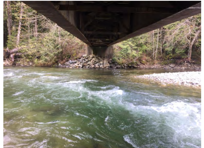
Right Bank Abutment when facing downstream
